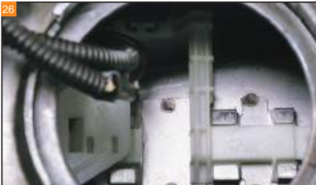
The stock components will lock in place inside the new tank.
